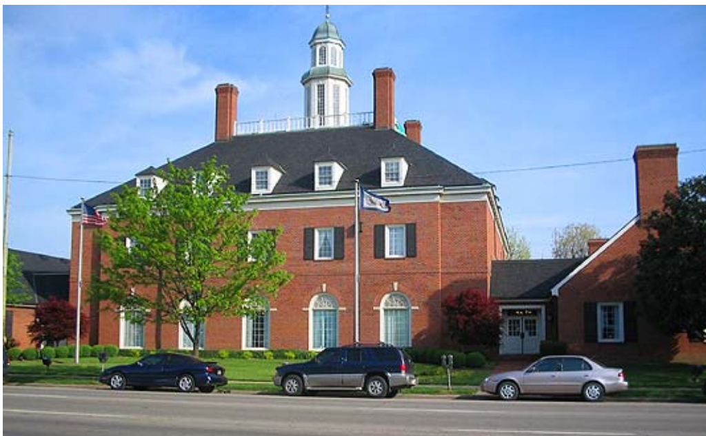
Marshall University's Center for Business and Economic Research is located at the corner of 3rd Avenue and 20th Street in Huntington, West Virginia in the City National Bank Building
