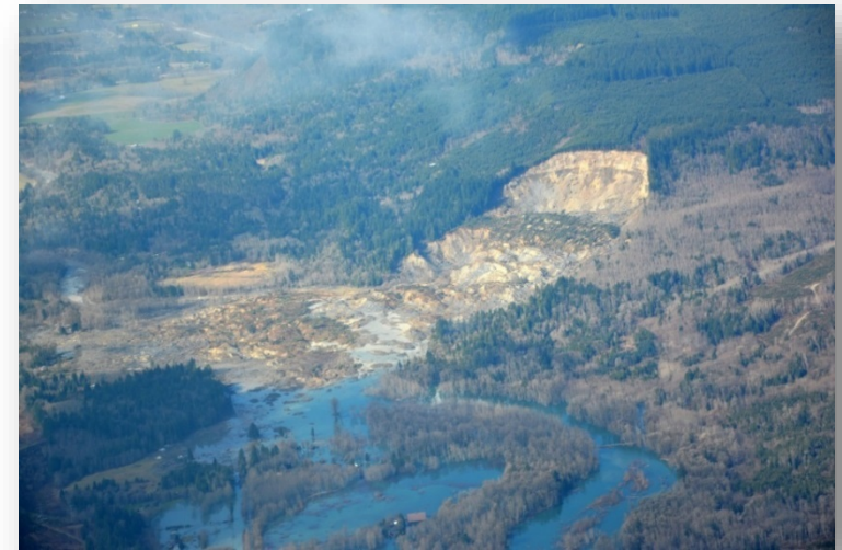
SR 530 Oso Landslide, Snohomish County, WA 41 life lost ((Source; Wash DOT)
