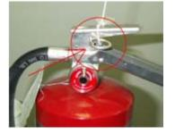
4. Visually inspect the hose and nozzle to ensure they are in good condition, showing no signs of cracking or dry rot.
