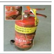
6. Check the inspection tag for previous and required inspection, maintenance, or charging and sign and date your inspection.
