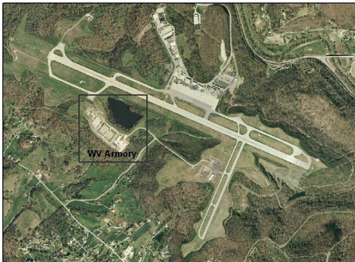
Figure 1: National Guard Armory
