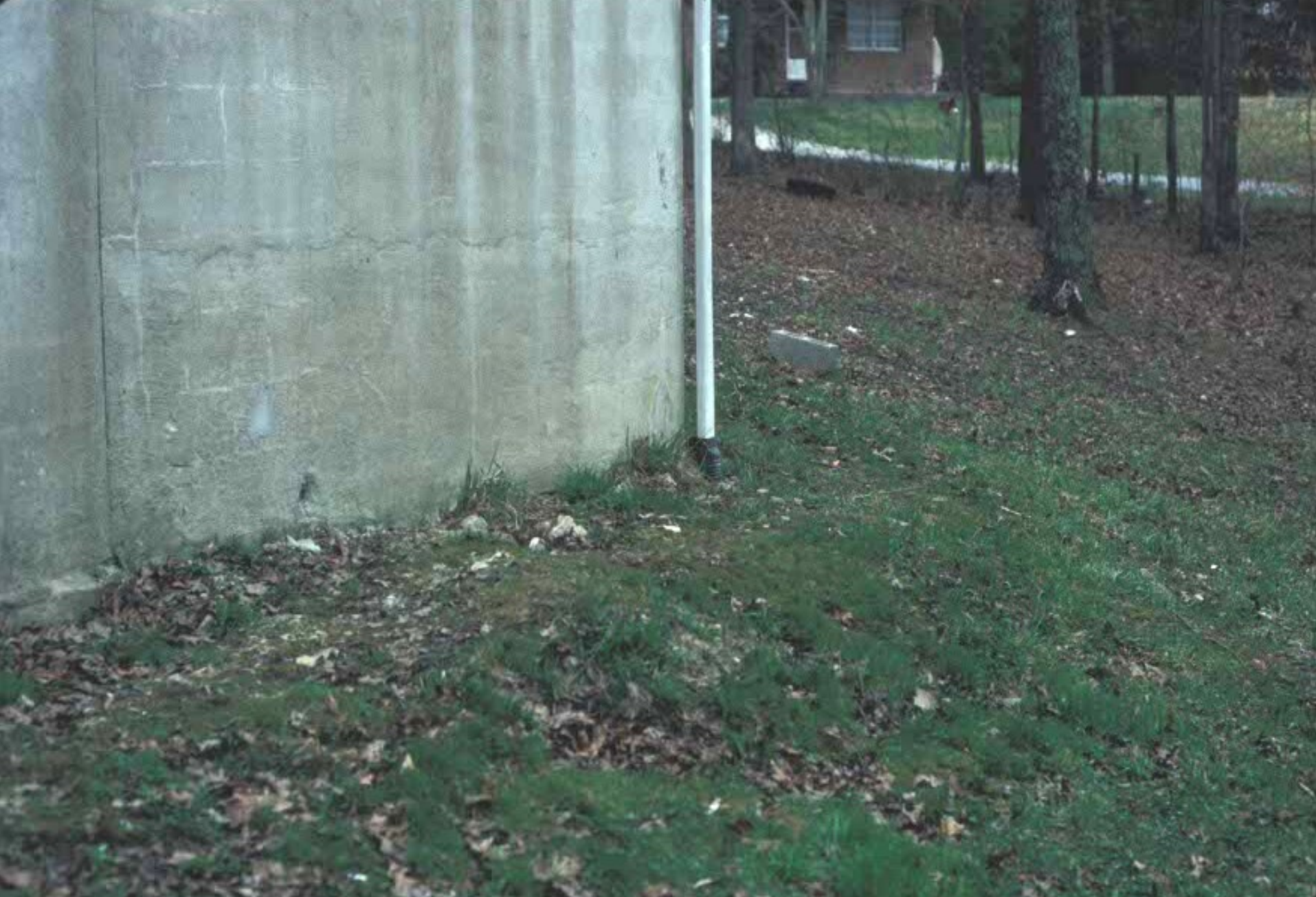
POWELL COUNTY – REAR CORNER OF HOUSE WAS PATCHED BECAUSE THE CISTERN BLEW UP. NATURAL GAS FROM THE SHALE WAS SEEPING IN
