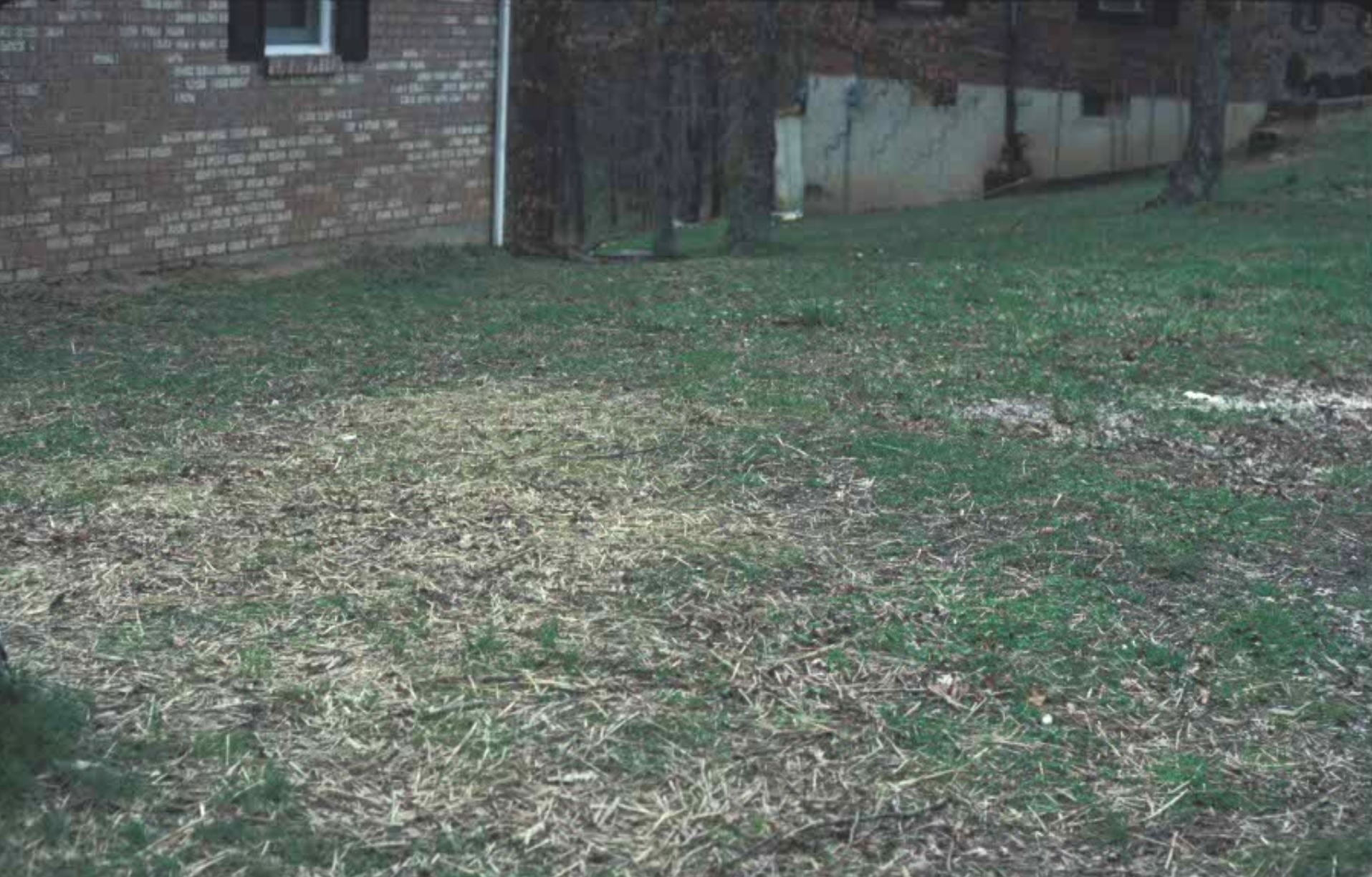
POWELL COUNTY – YARD SLOPED DOWNWARD FROM ROAD ALLOWING WATER TO BUILD UP AGAINST HOUSE AND SEEP UNDERNEATH. NOTE CRACKS IN NEIGHBORS HOUSE.
