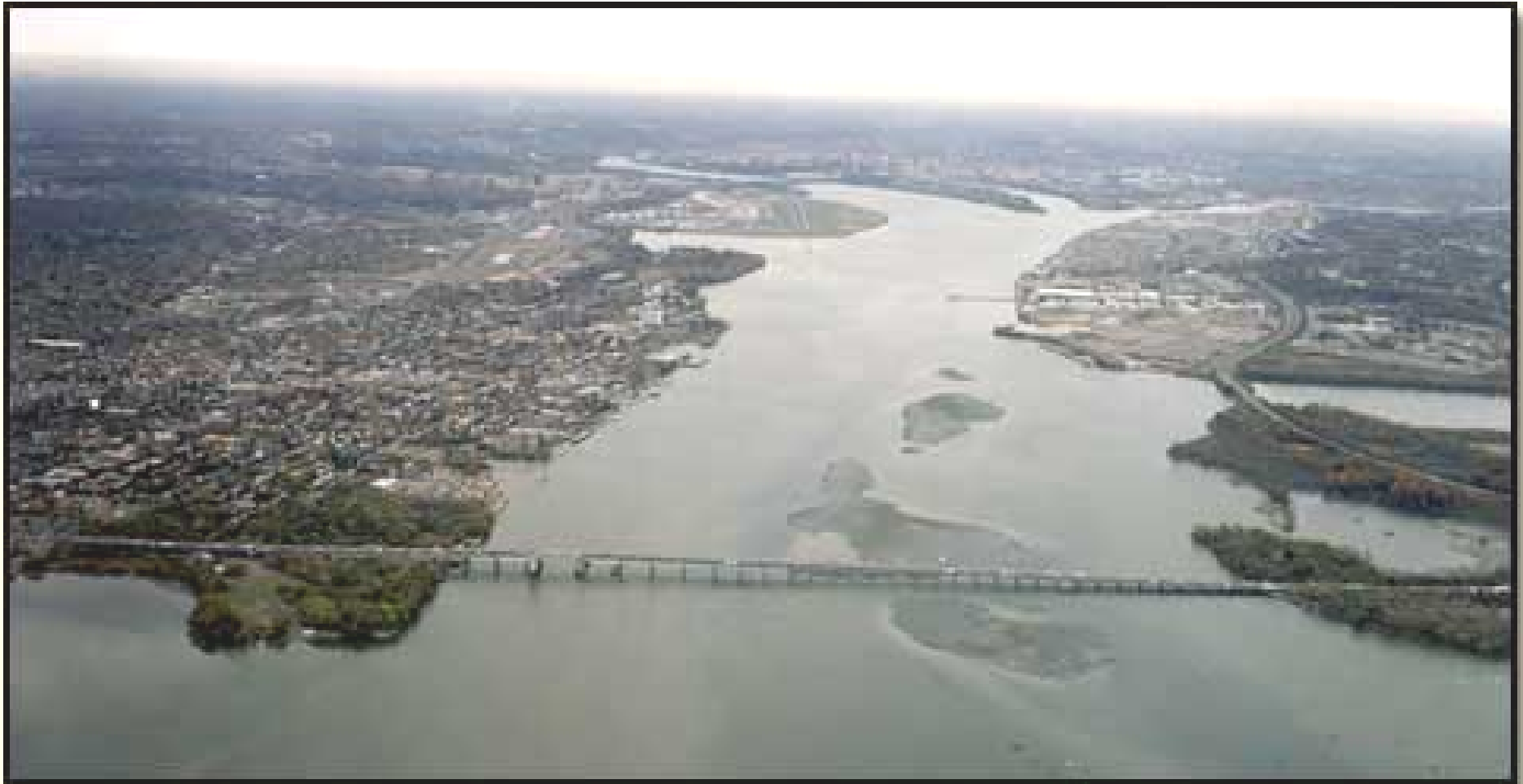
Aerial Photo of Existing Woodrow Wilson Bridge
