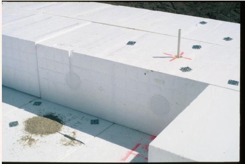
Magnet Extensometer and Pressure Cell Installation
