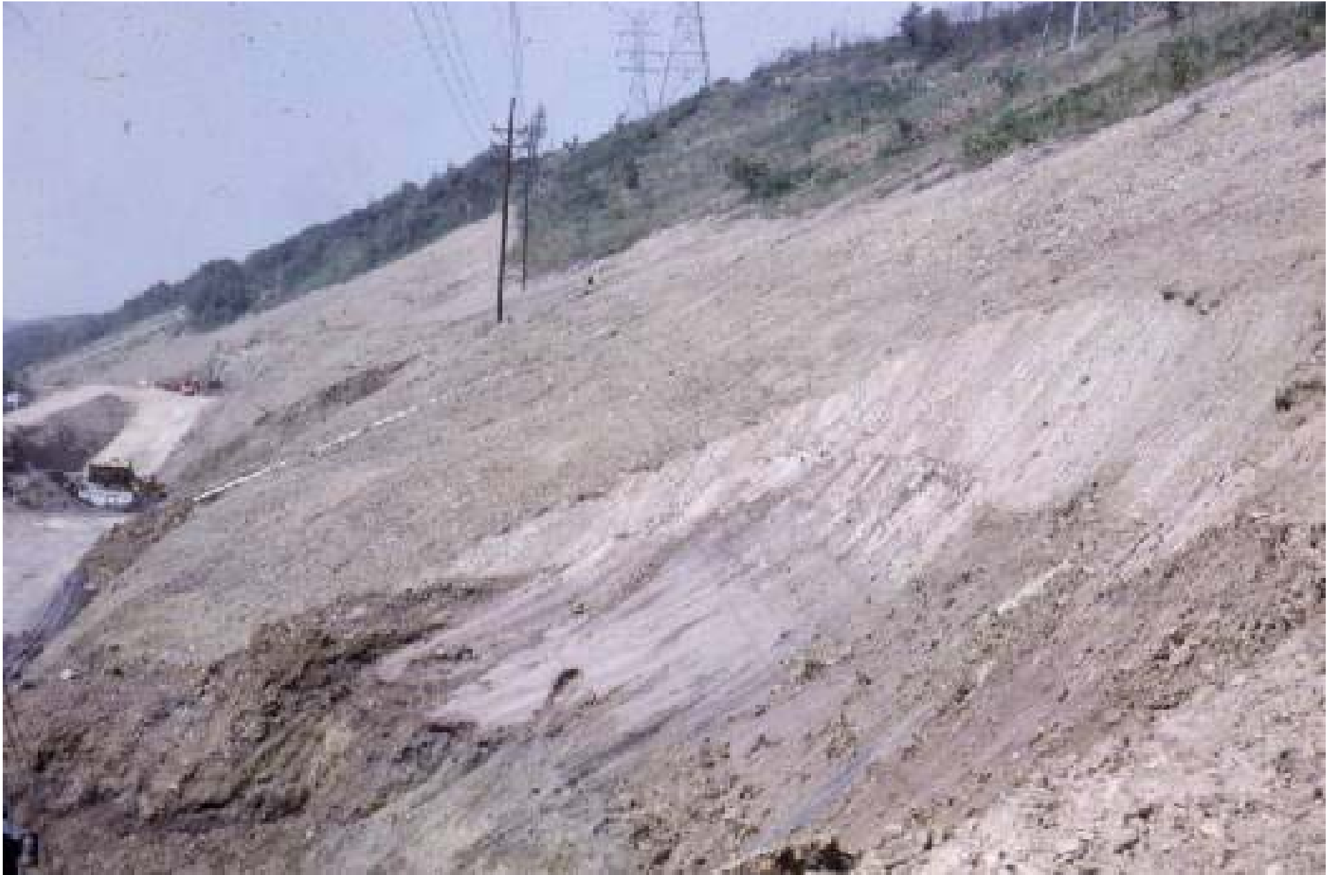
EXPOSED MOVEMENT SURFACE IN A COLLUVIAL SOIL WEIRTON, W. VA
