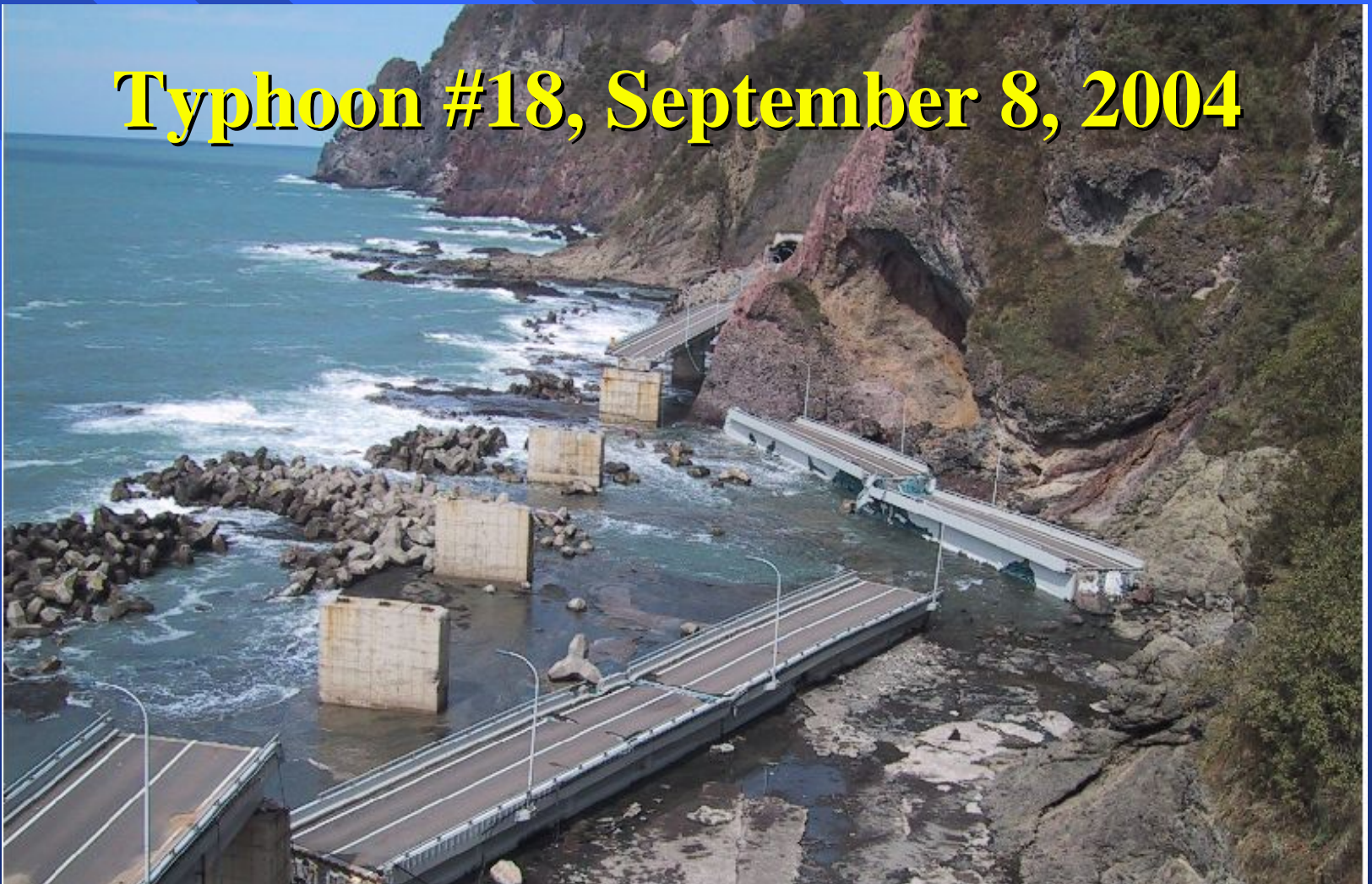
The Ohmori-Ohashi Bridge – Hokkaido, Japan
