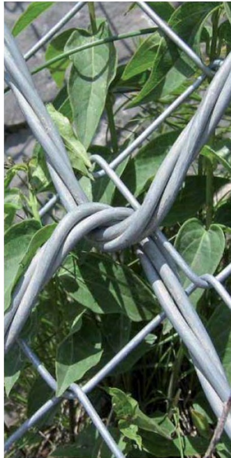
Mesh to Mesh Connection - Single Twist
