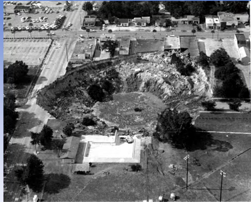
Winter Park, Florida sinkhole in 1981 (~320 ft. wide, ~90 ft. deep)
