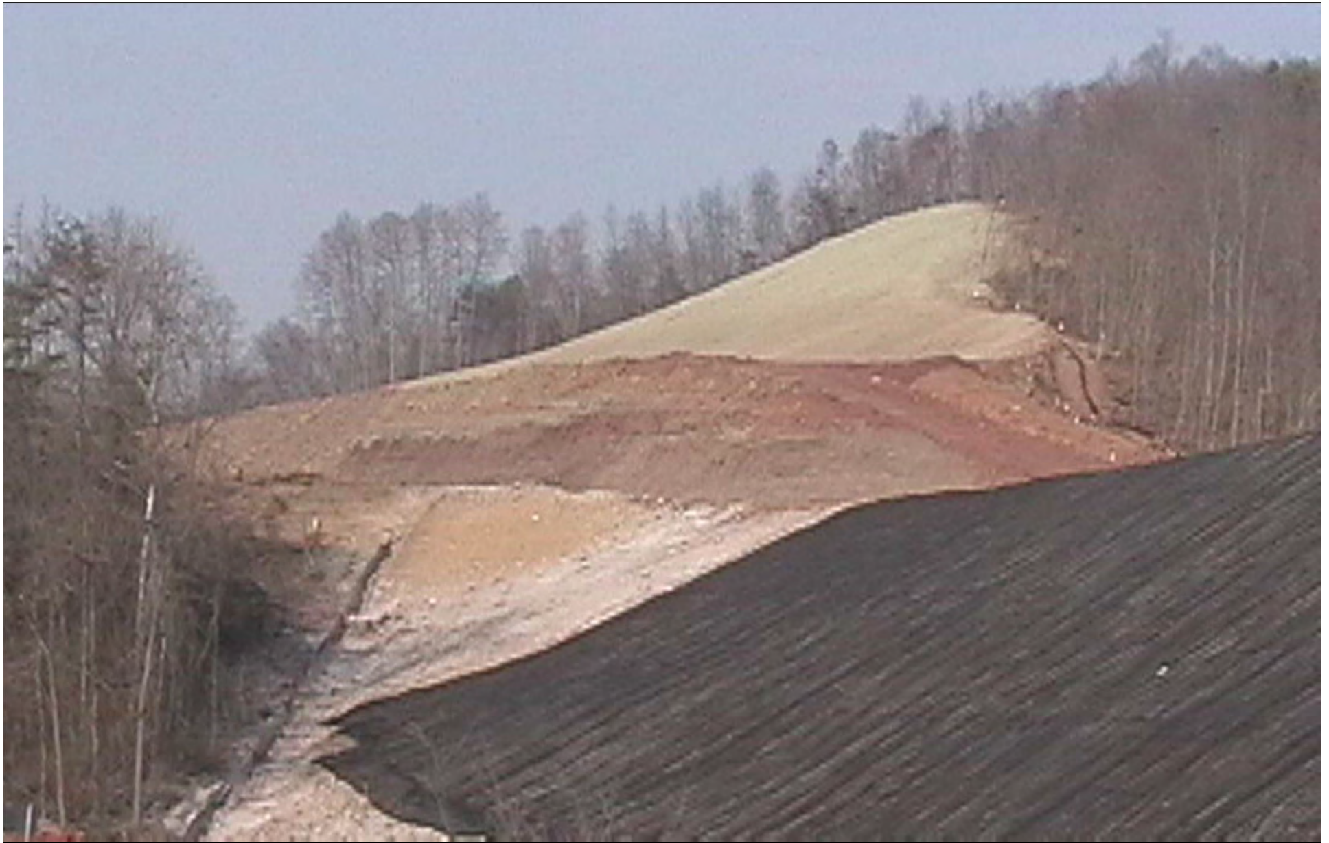
Constructed Reinforced Soil Slope
