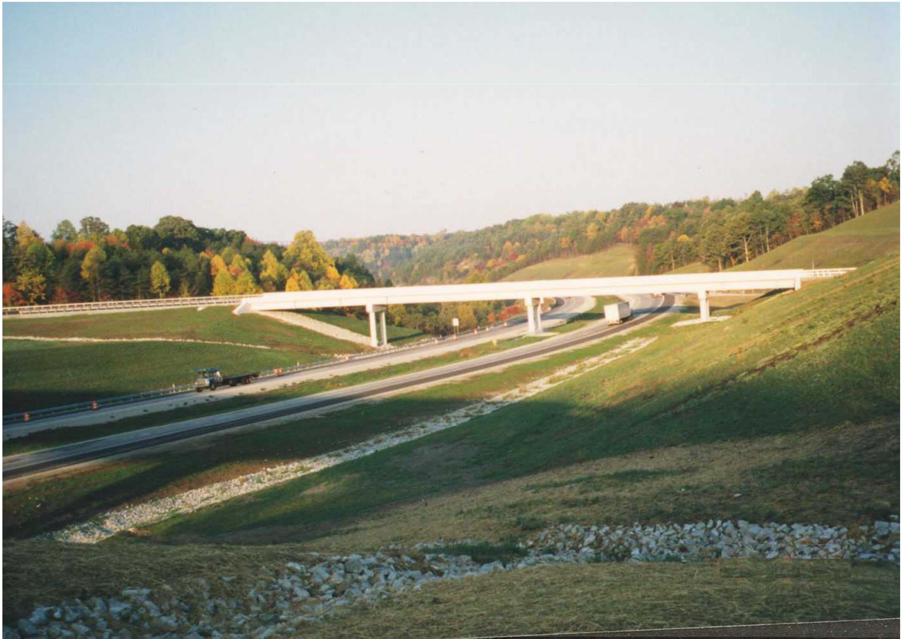
Industrial Parkway / I-64 Interchange
