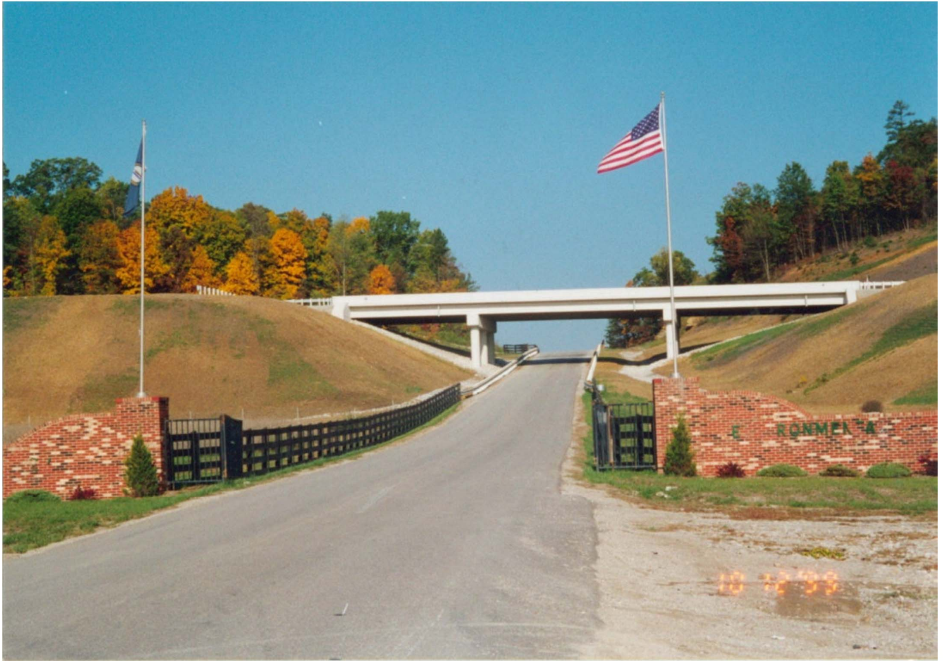
View of Approach Embankment after Construction
