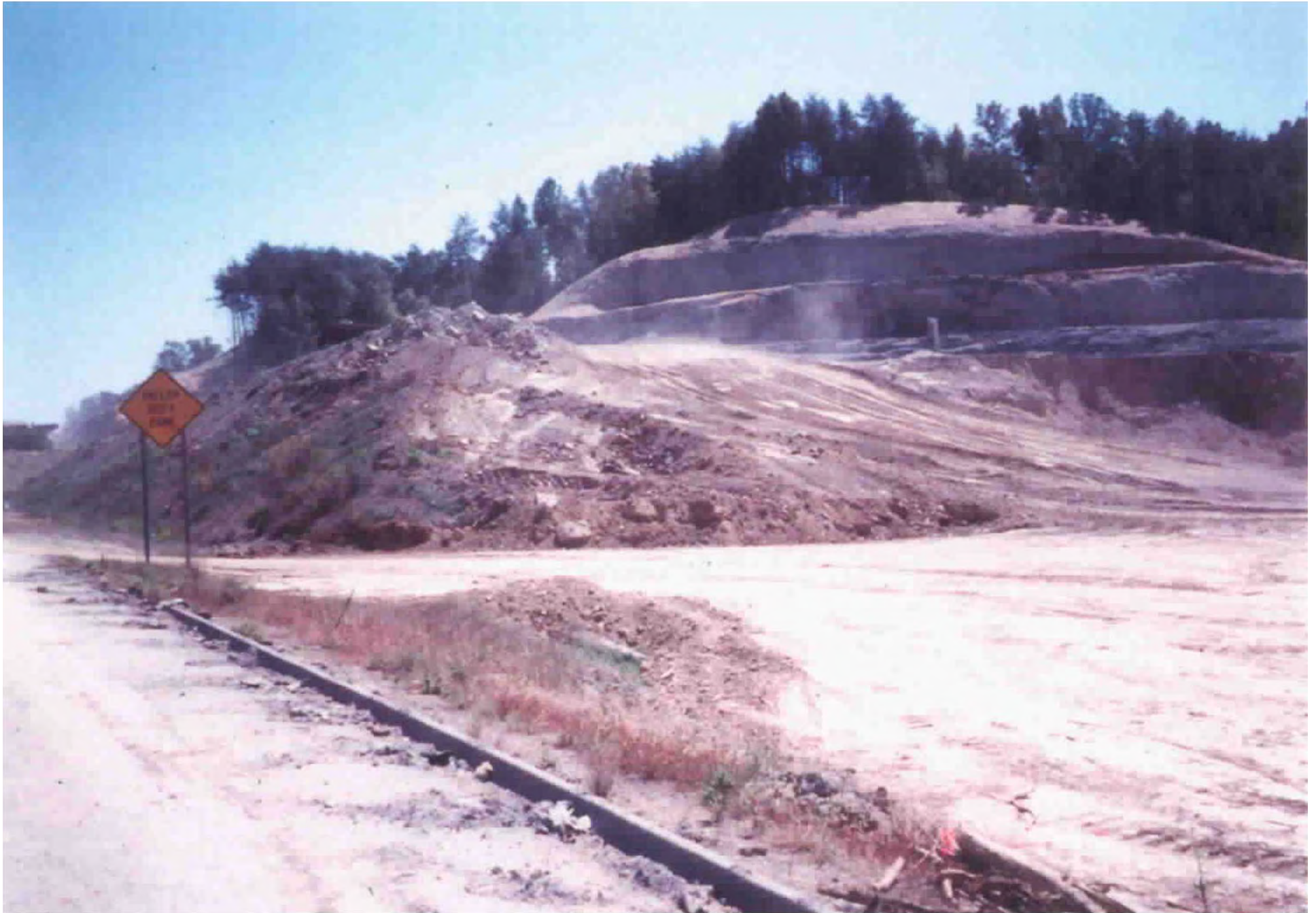
Roadway Cut being Constructed within Non-Durable Shales
