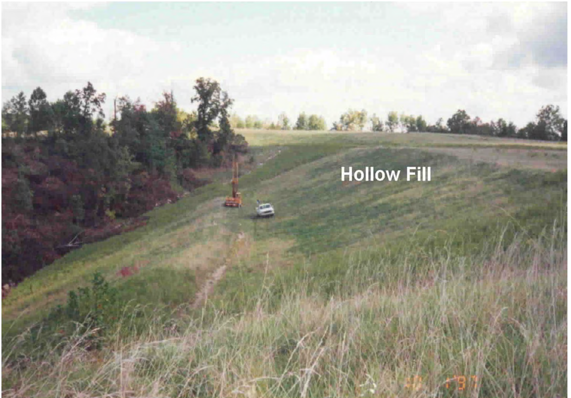
Typical Hollow Fill Encountered Along the Project
