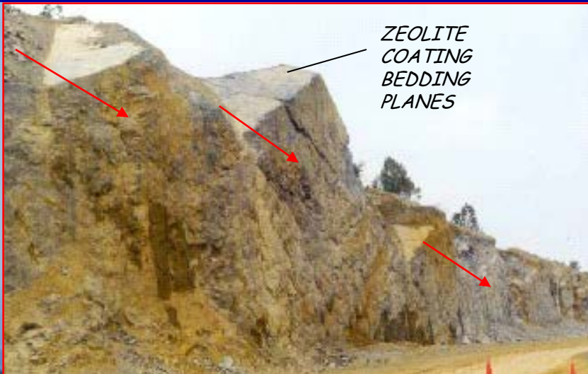
Smart Road Deep Cut Looking Southwest "Highly Unstable"
