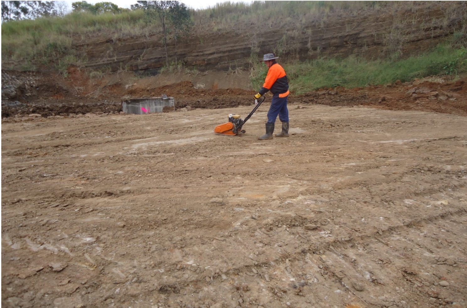
Compacted fill after the third geosynthetic layer
