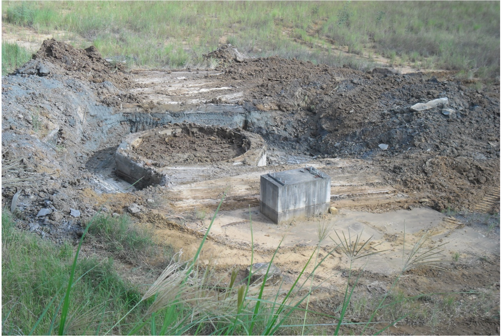
Exposed air shaft looking South
