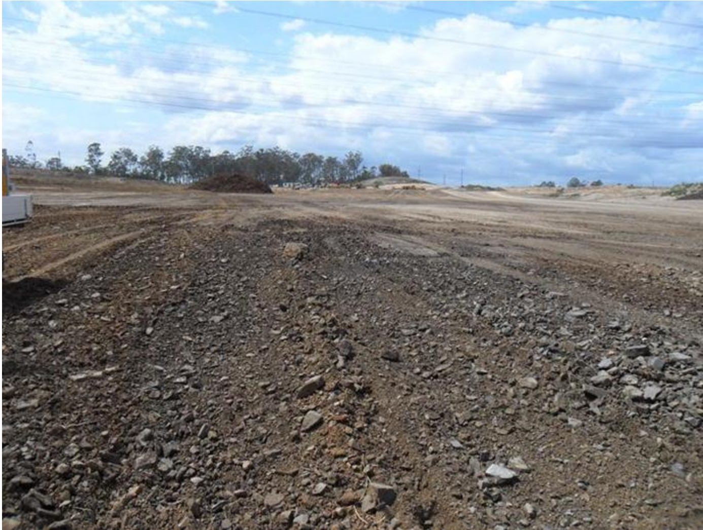
Compacted backfilled sinkhole area
