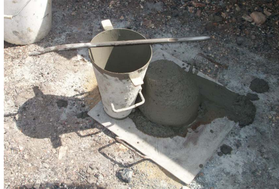
Slump Test on Barrier Grout (6 in slump)
