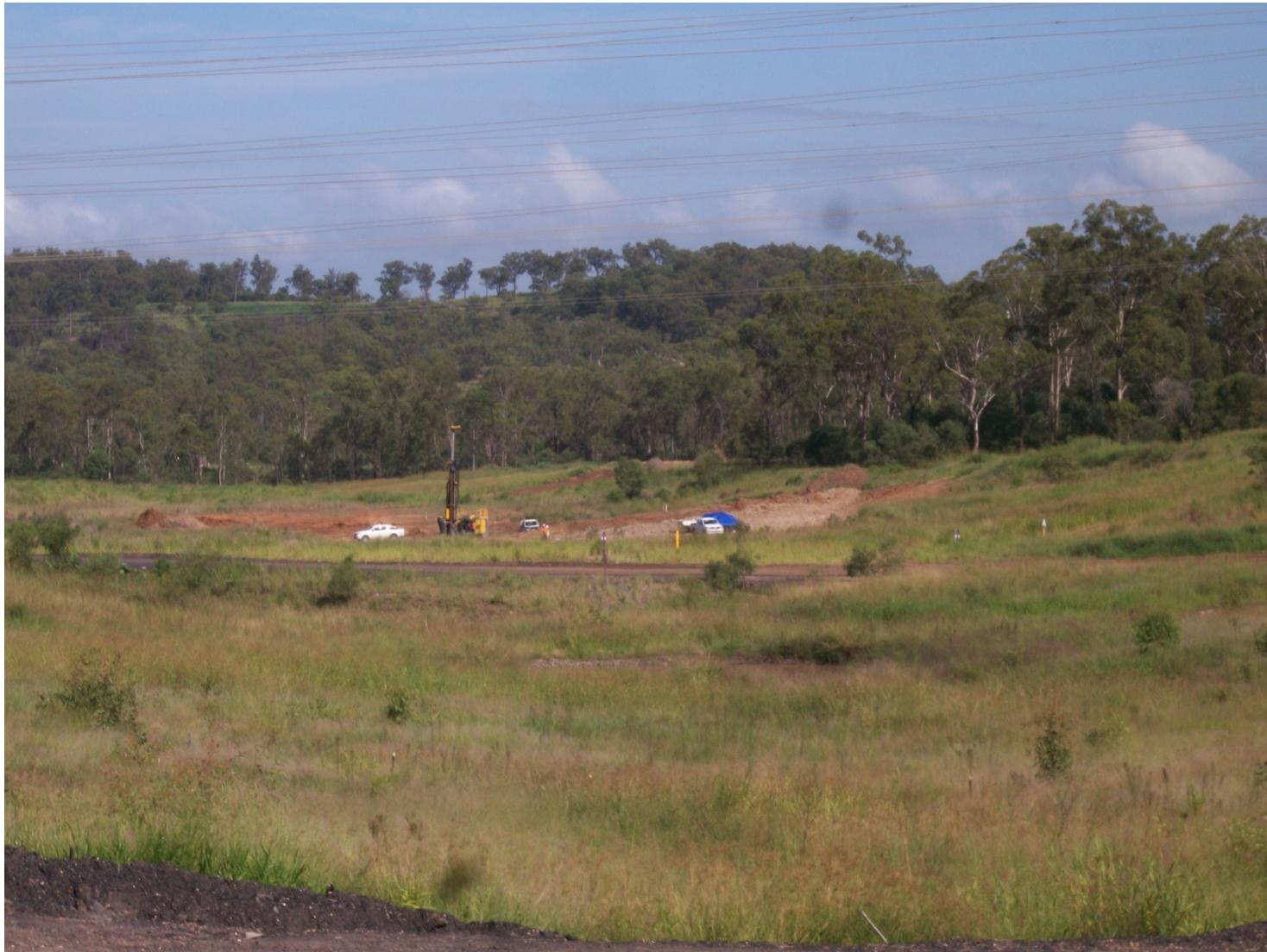
Overview of drilling area
