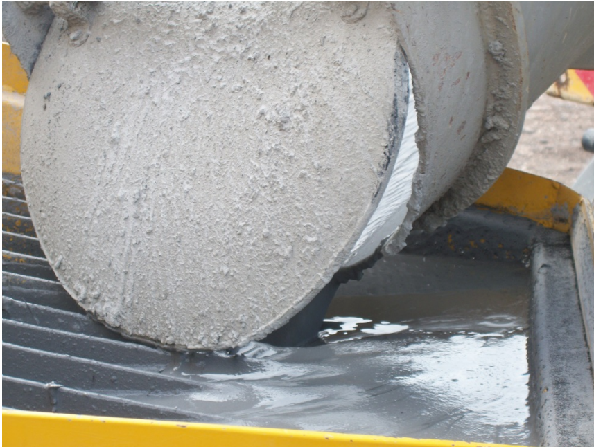
Infill Grout in Hopper (25 – 35 Sec Flow Cone)
