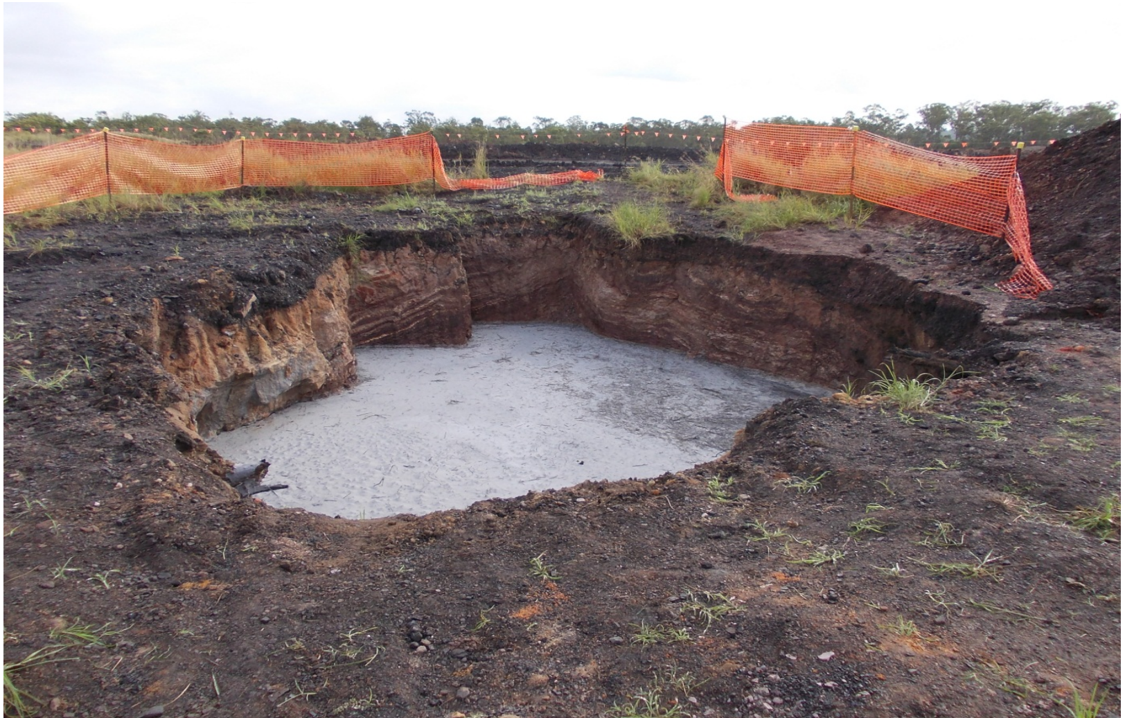
Tunnel 2 after filling with grout
