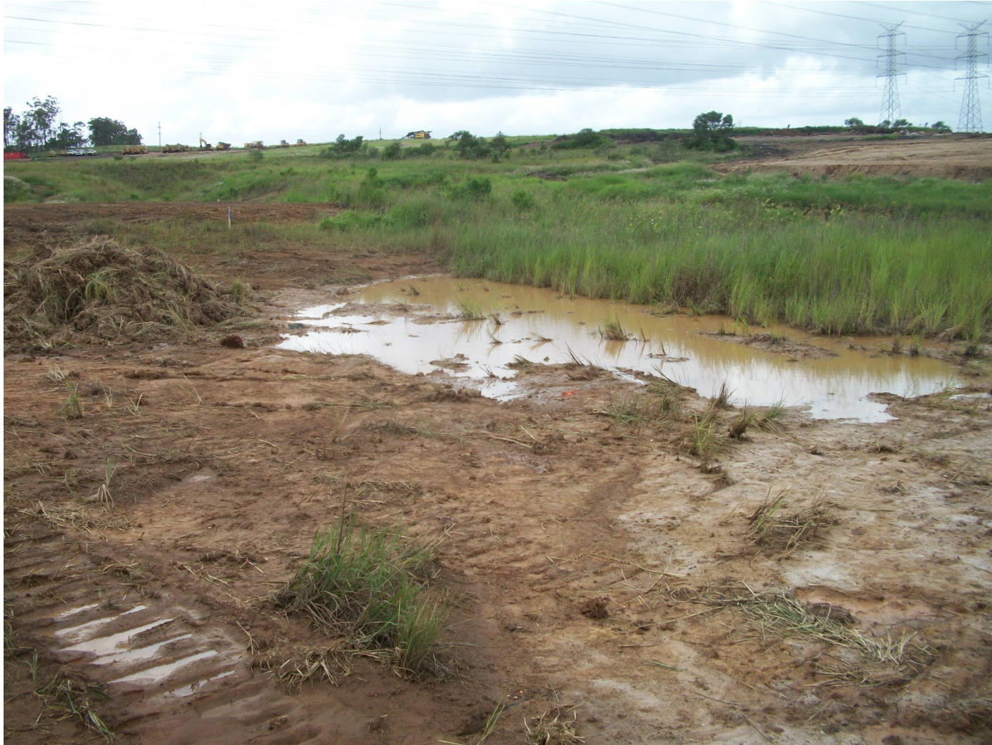
Backfilled sinkhole area at Belt Tunnel prior to drilling
