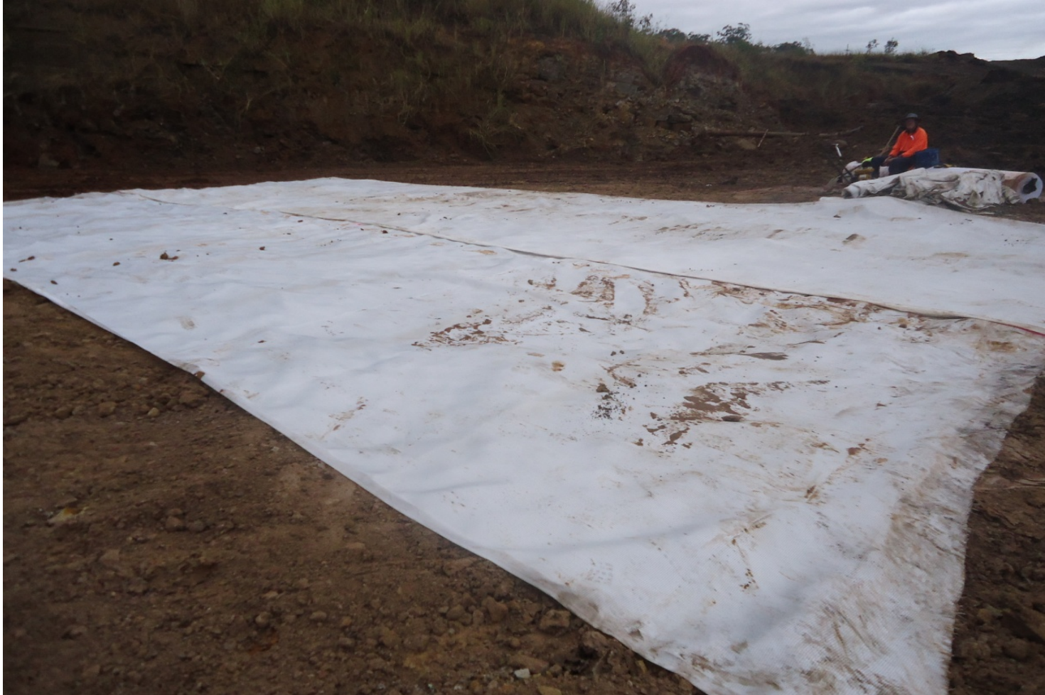
First geotextile layer spread over shaft
