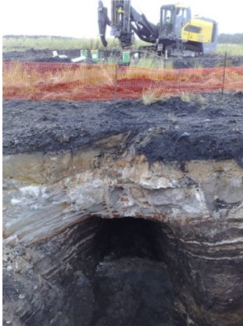
Grout hole drilling
