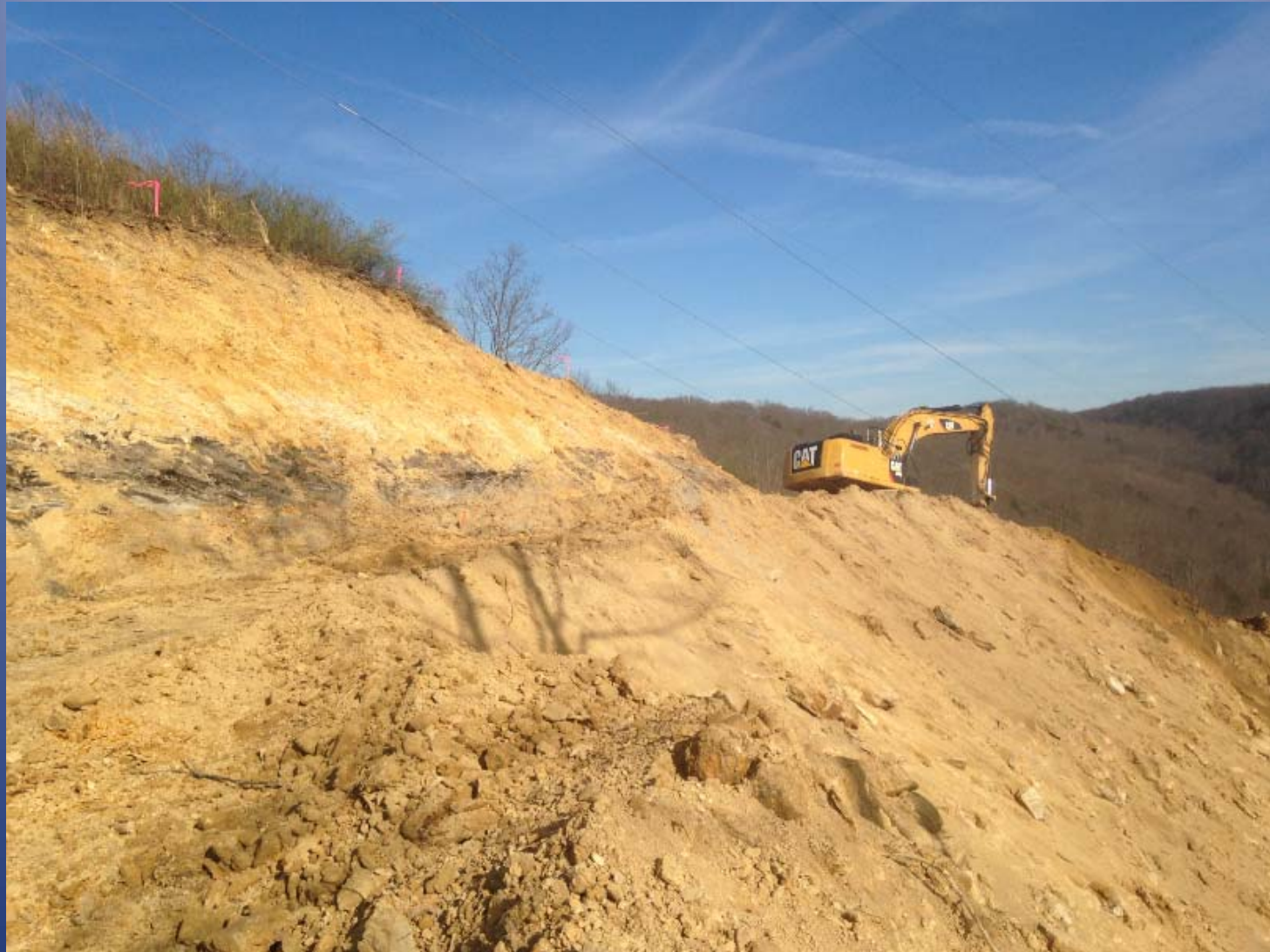
March 8, 2016, excavation of shaly clay at top of slope
