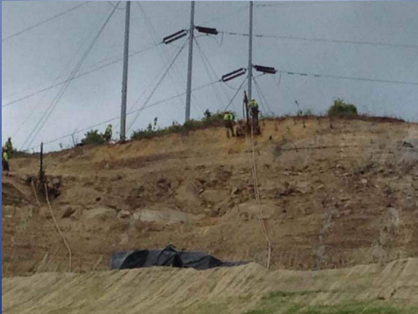
Installation of nails in shaly clay, note closer spacing
