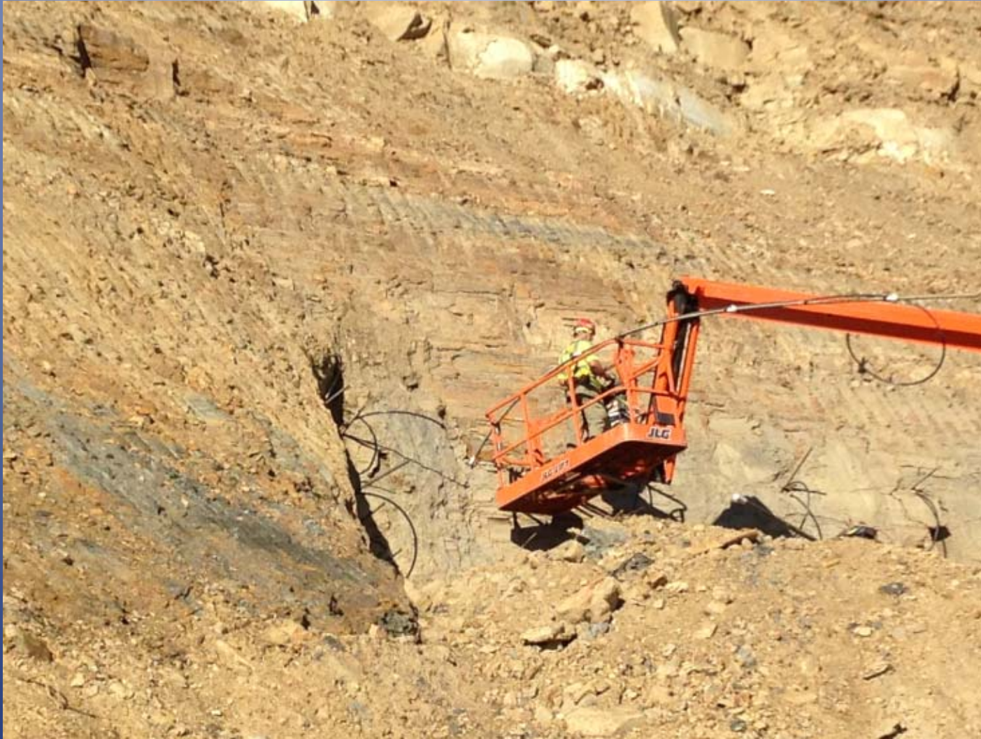
March 28, insertion of anchors for combination shotcrete/wire mesh covered slope
