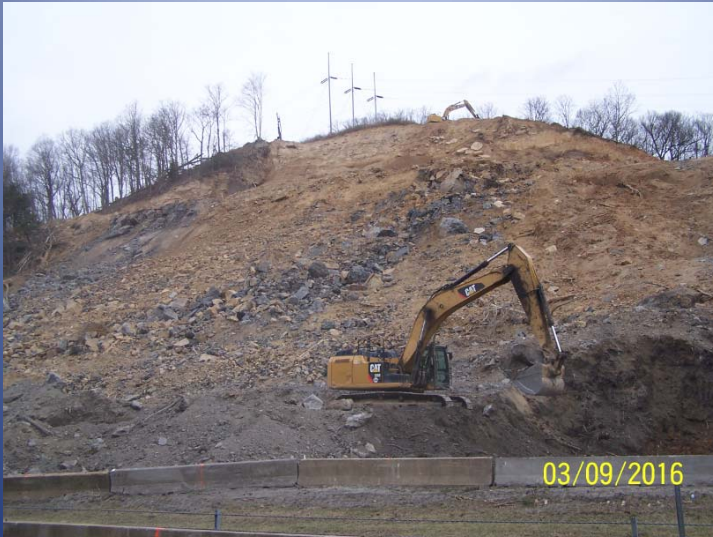
Debris removal continues
