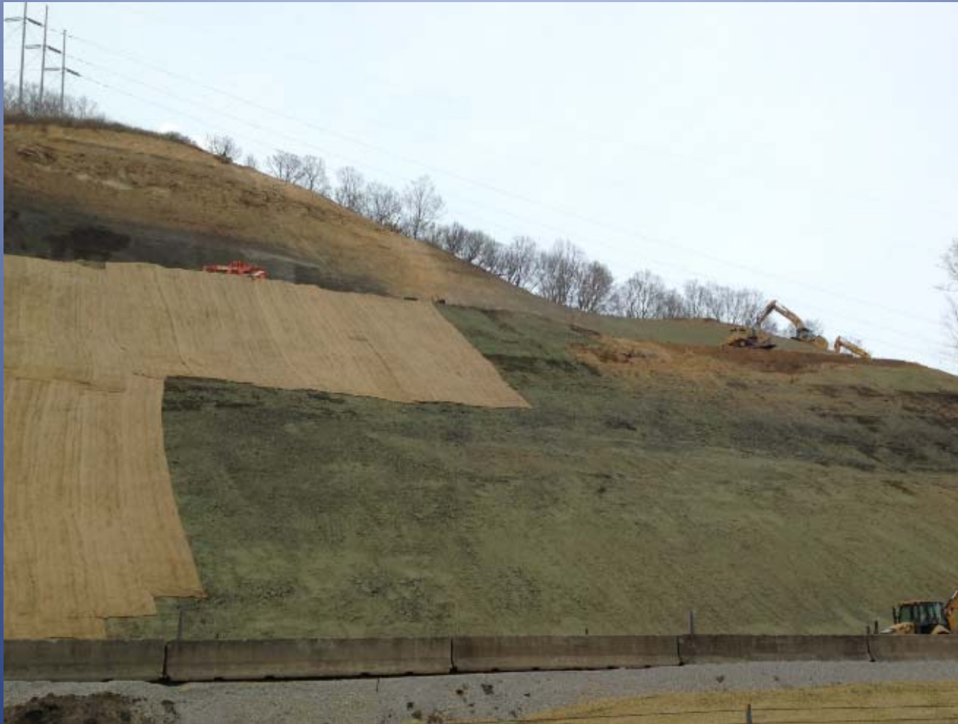
Removal of slide debris from lower slope nearing completion April 13, 2015
