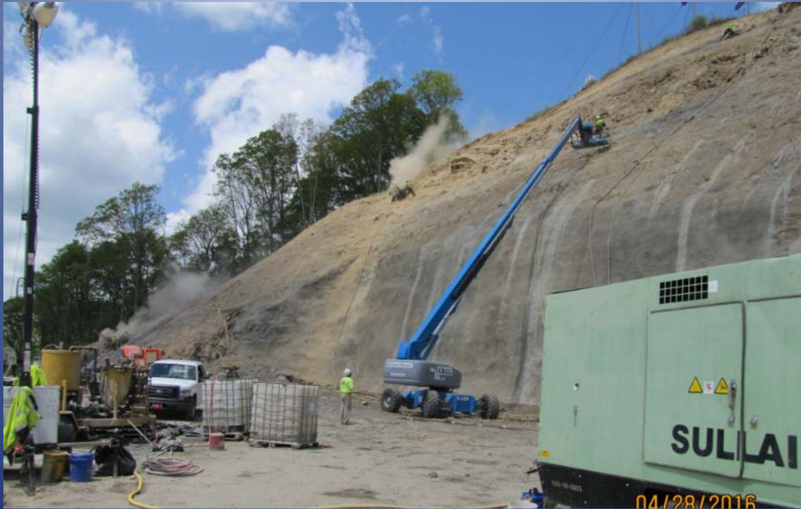
Drilling for anchors in upper 1:1 slope
