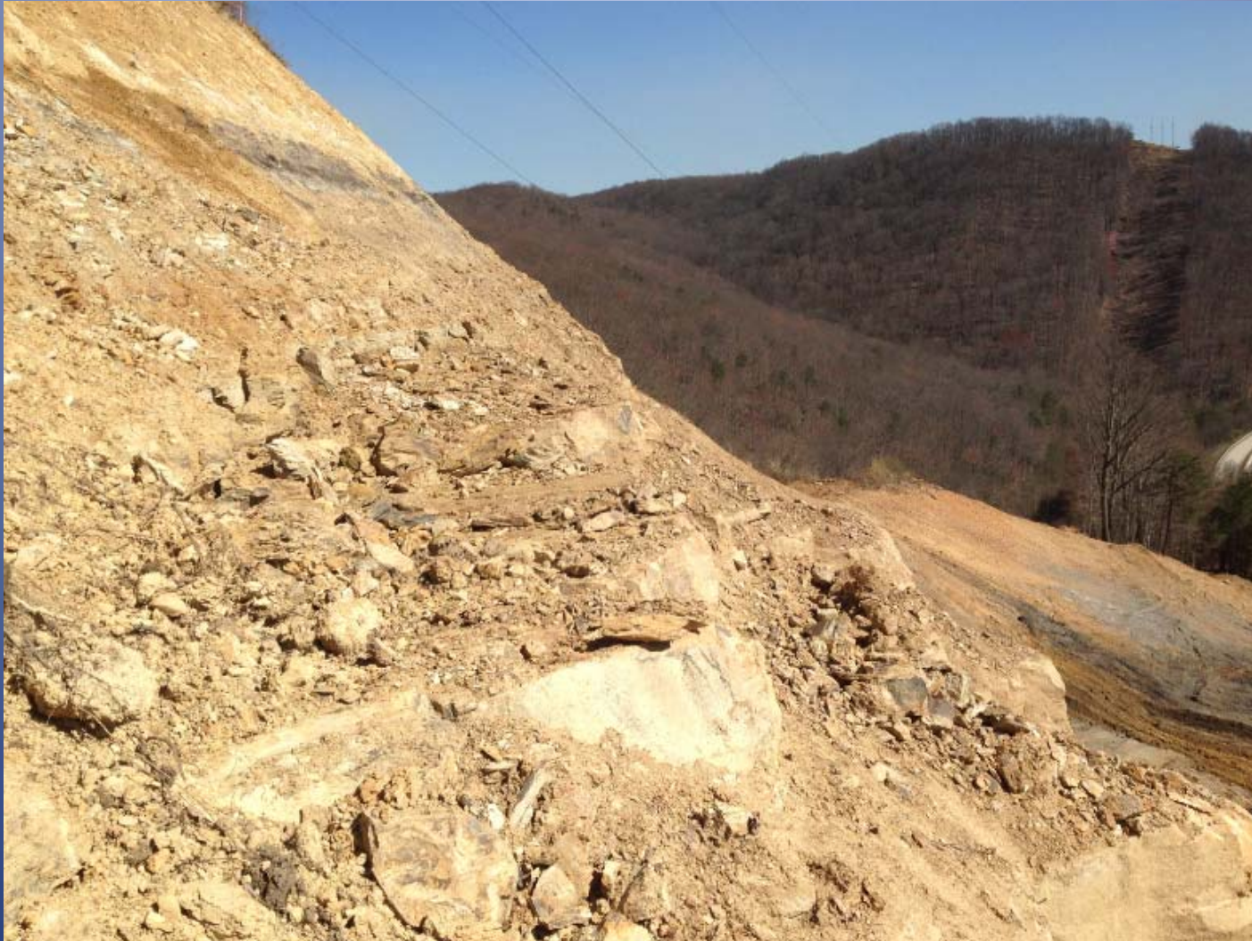
Sandstone layers near top of slope, note dip of strata
