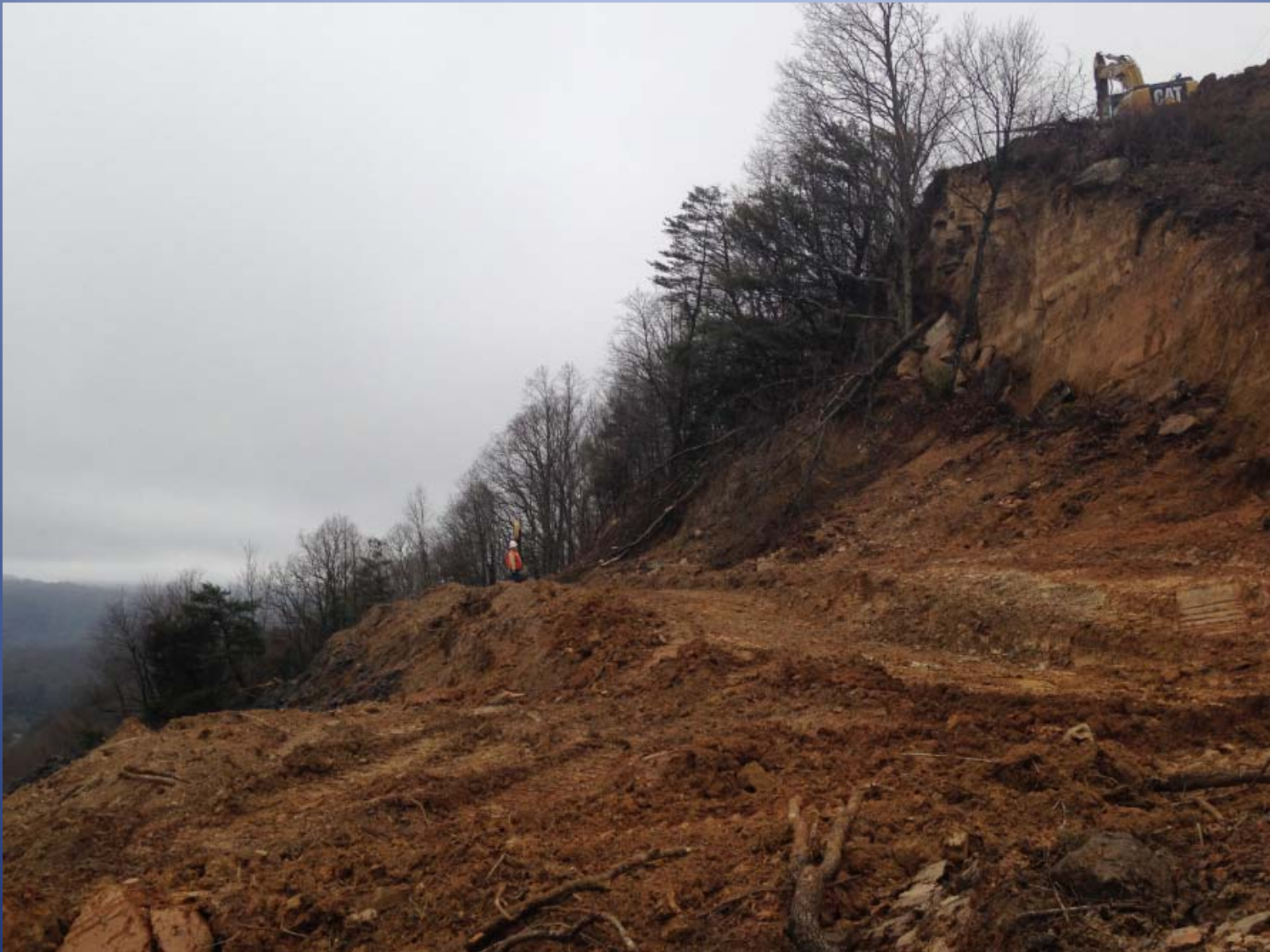
March 4, 2016 - Removal of slide debris from slope
