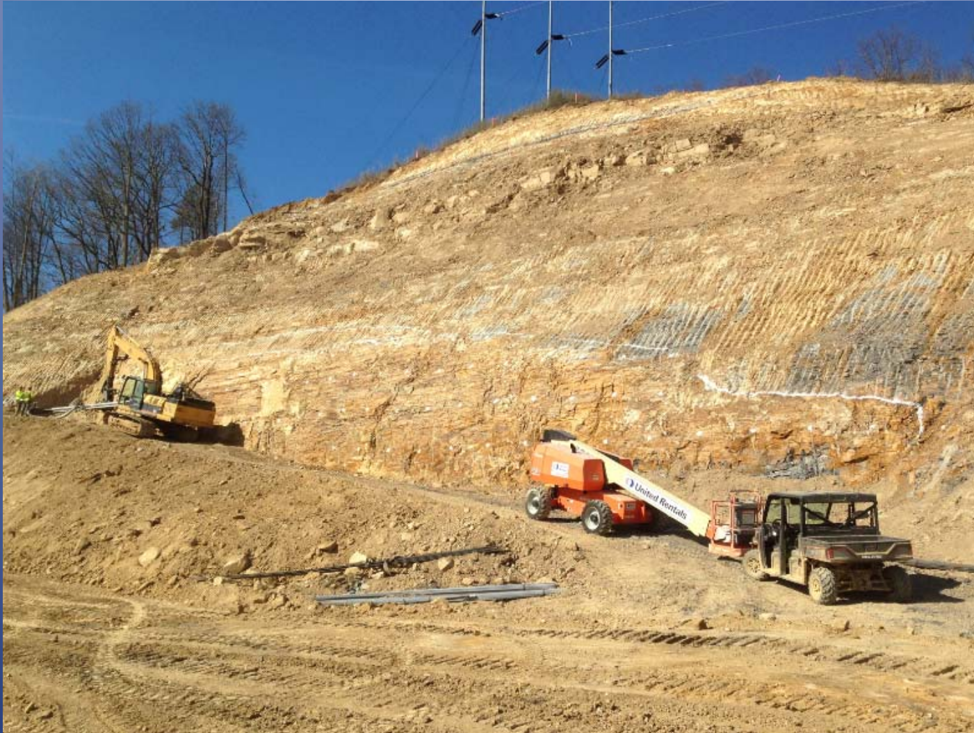
Preparing to anchor and shotcrete lower slope 3/23/16
