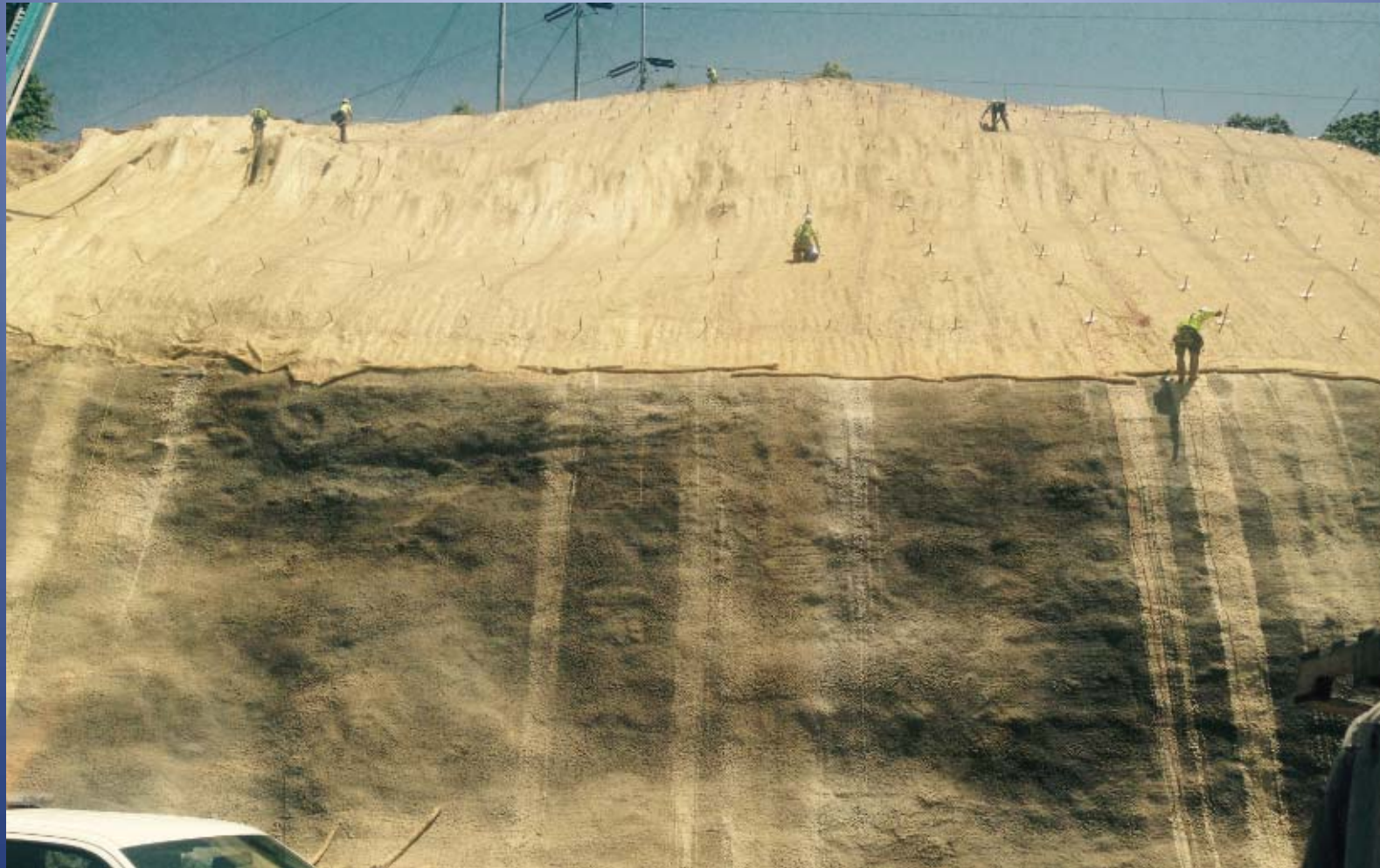
Placement erosion control matting prior to placement of wire mesh, May 23
