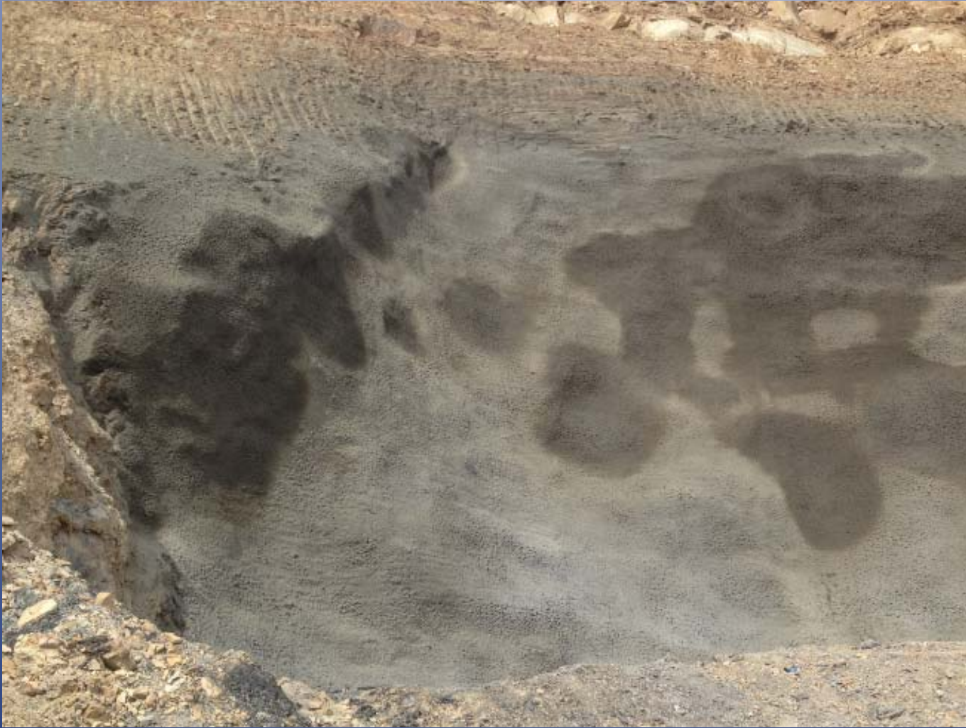
Slope after shotcrete application
