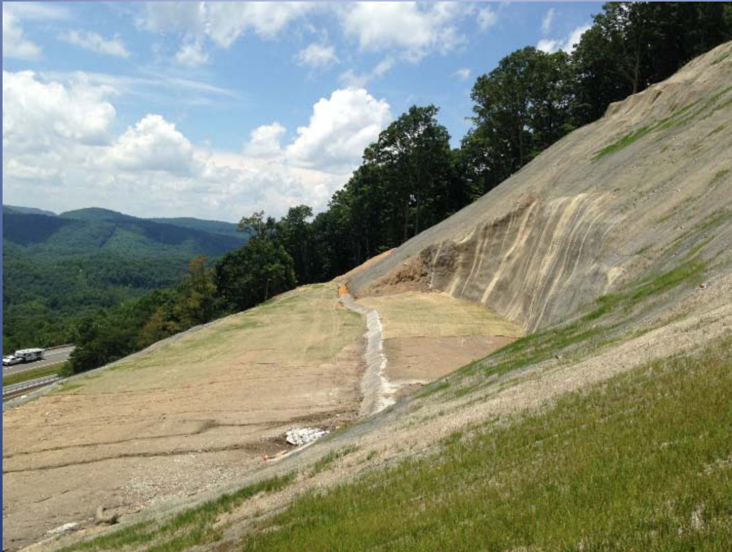
Grade Beam in Place
