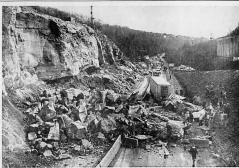
Scene of rockslide on Saw Mill Run Boulevard, between Fort Pitt and Liberty tunnel entrances. Two people were killed and one injured when boulders tumbled from hillside.
