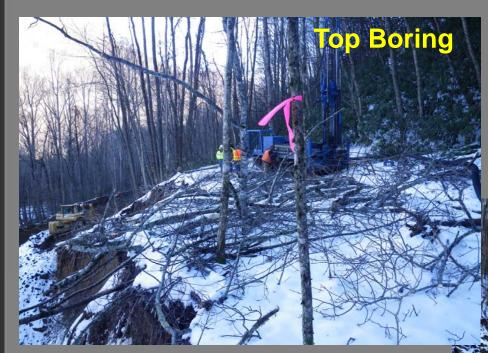
Borings drilled at the top and bottom of failed slope
