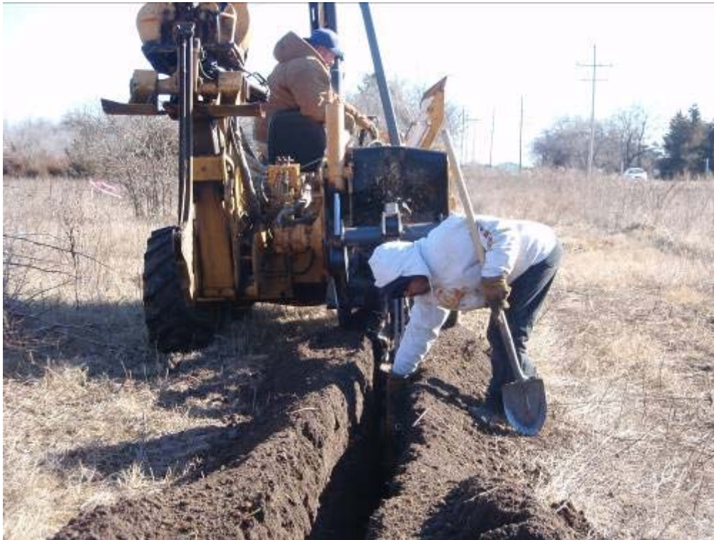
Digging of the trench where the sensor is deployed
