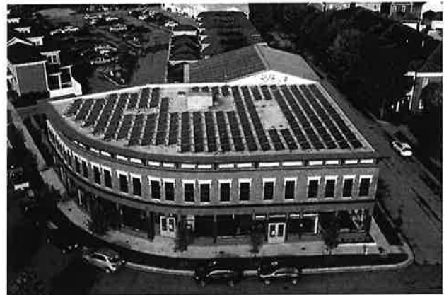
CMTA Energy Solutions Corporate Office Louisville, Kentucky
