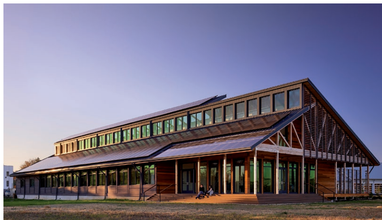
Below: Semans-Griswold Environmental Hall at Washington College , designed to operate at net-positive energy and to meet the holistic standards of Living Building Challenge Petal Certification.
