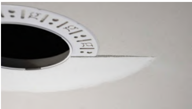
Partially finished mud ring, showing cross-section detail.
